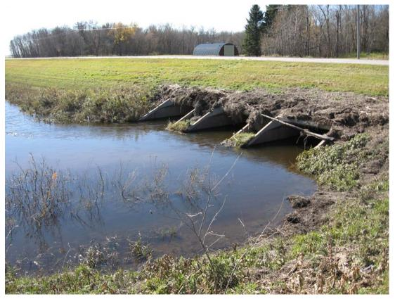
Debris piled on top of the culverts at the Hwy 54 crossing of the Moose River, indicating how high the water got in September.
